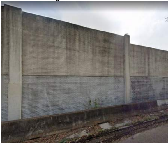
Existing Concrete Noise Wall
