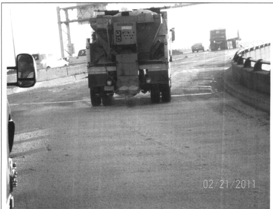
AI#:175084 Date: 2/21/2011 Description: Sanding the On-Ramp
