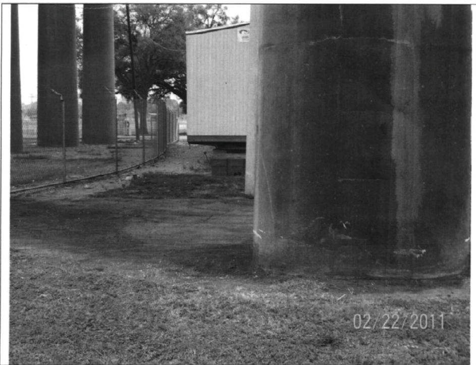
AI#:175084 Date: 2/22/2011 Description: Remediated Area
