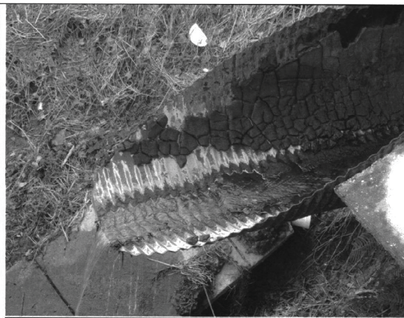
Photo #: 6 of 10 Time: 9:10 AM Description: Pipe the affected water comes out of – pinkish hue; seen in pipe.
