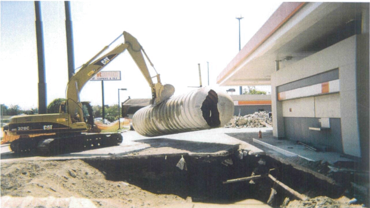
PHOTOGRAPH 2: 10,000-gallon gasoline or diesel fiberglass UST following removal.
