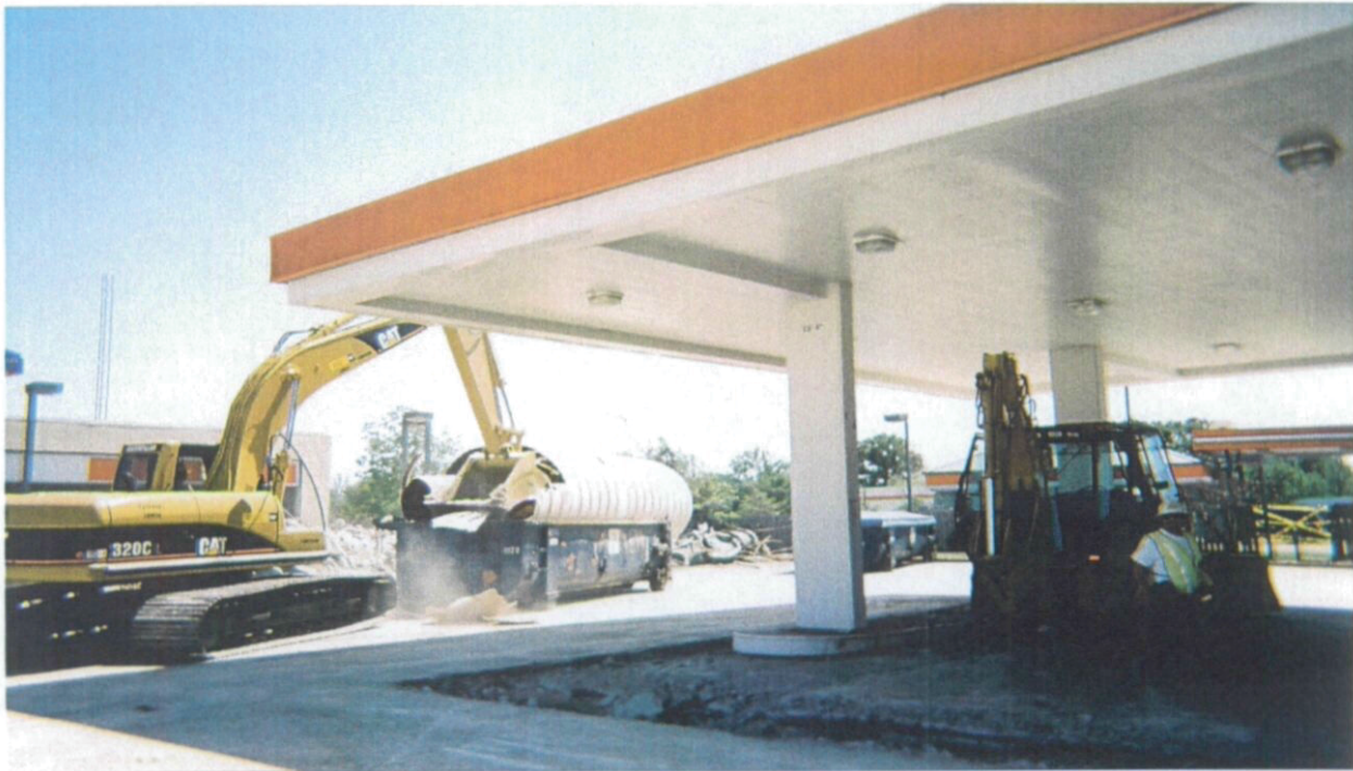
PHOTOGRAPH 3: 12,000-gallon gasoline fiberglass UST being destroyed.
