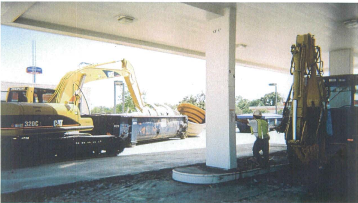
PHOTOGRAPH 4: Fiberglass USTs being destroyed.
