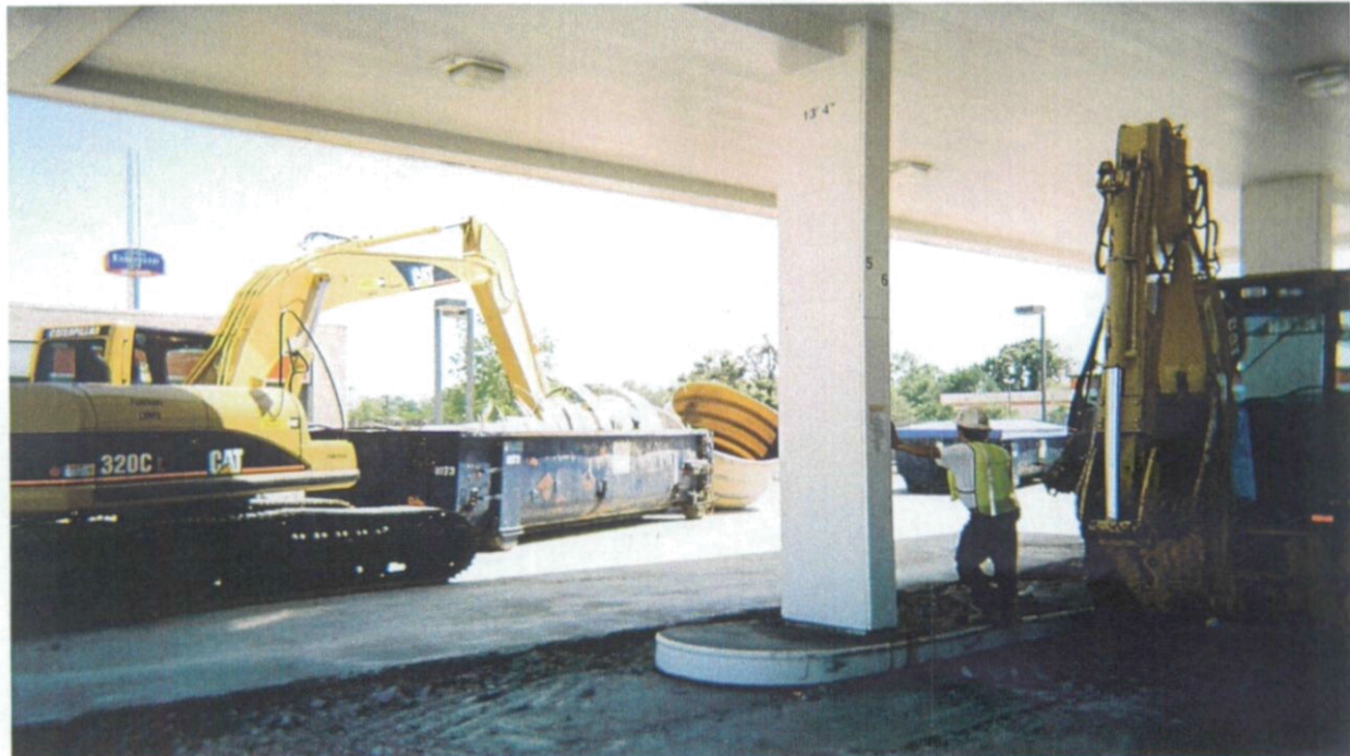
PHOTOGRAPH 4: Fiberglass USTs being destroyed.
