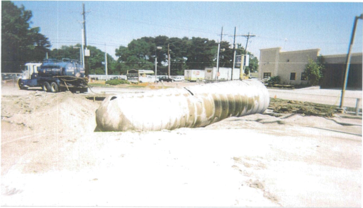
PHOTOGRAPH 1: 10,000-gallon diesel or gasoline fiberglass UST prior to removal.
