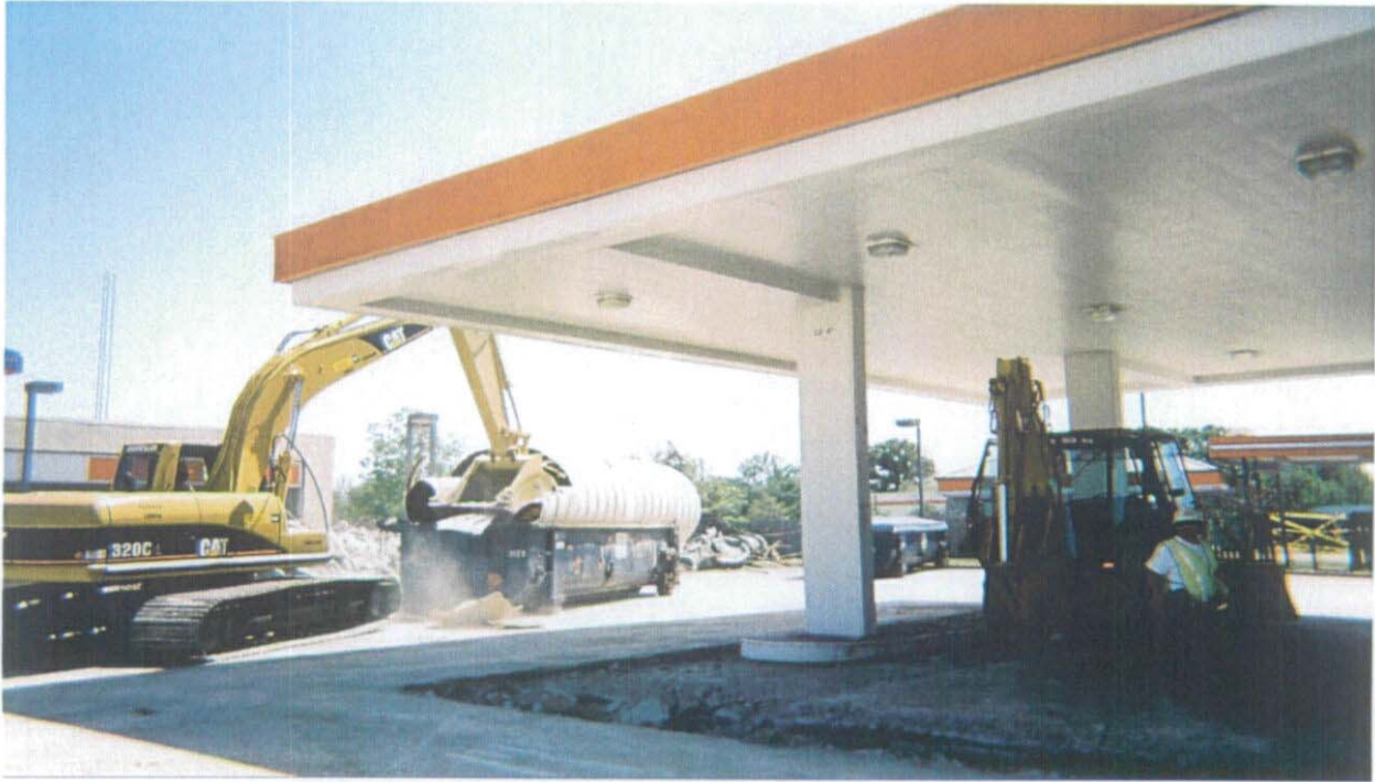
PHOTOGRAPH 3: 12,000-gallon gasoline fiberglass UST being destroyed.
